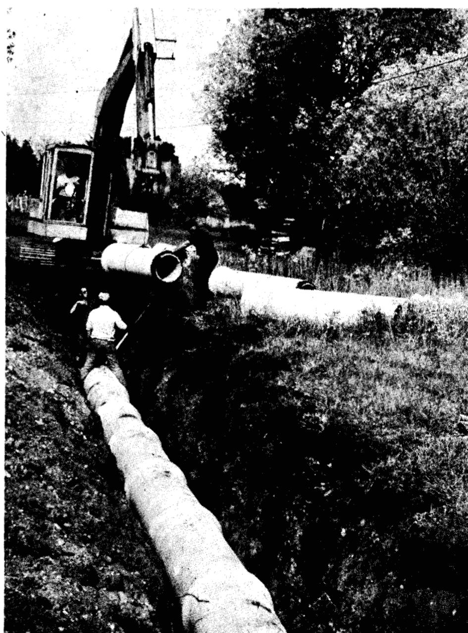
CONSTRUCTION WORK has begun on the senior citizen housing project at the end of Woodland St., Cass City. Last week workers began installing sewer lines for the 24-unit complex.
