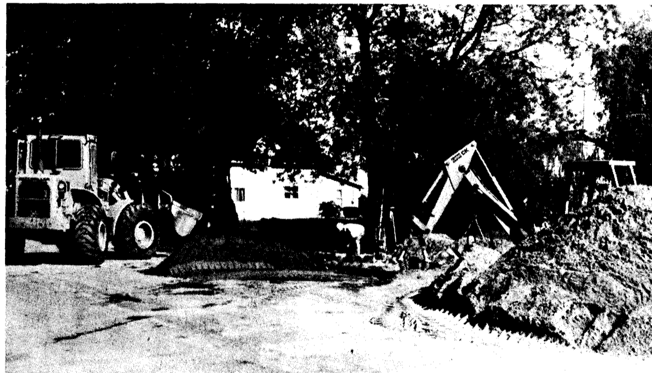
CONSTRUCTION WORK on the Owendale sewers is on schedule with the main lines to be completed soon and the work on the lagoon to be completed by November. Individual hookups are scheduled to begin next spring.
