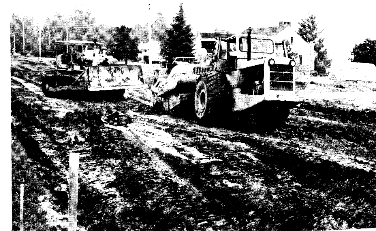
REBUILDING of the two-lane portion of N. Seeger Street into four lanes is continuing, with completion scheduled before the start of school. Completion was delayed due to discovery of some soft ground, which had to be removed and replaced with fill. The road will be more level in front of the high school.
