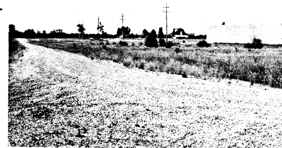
READY AND WAITING -- The industrial park along Doerr Road, owned by the Cass City Industrial Development Corp., has streets, sewer and water lines installed, ready for any company that wants to build a factory there.
