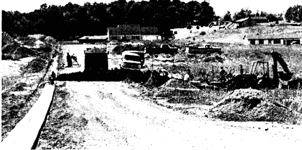
CURBS are being installed in the Northwoods Village subdivision in preparation for paving.
