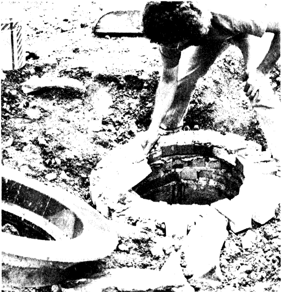
ALMOST DONE - Raising of this manhole on Sherman Street, done Monday, marked the end of construction of the sewer line extension and sewage lift station in the southeast corner of Cass City. Smoothing the cement was Karl Zawilinski. Some electrical parts, not yet delivered, must be installed, and testing and grading done before homeowners can have their homes connected to the sewer lines. Deadline for completion is July 31. Contractor for the $62,579 project is Andrew Barnes Jr.
