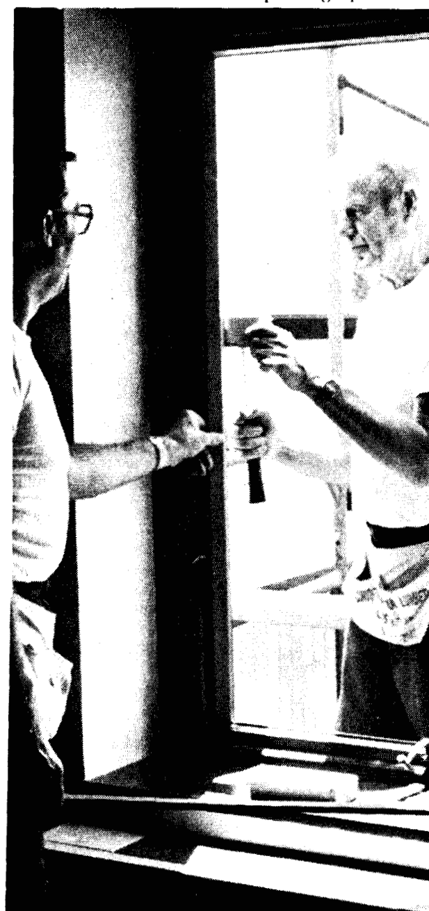
NEW WINDOWS are being installed in patients' rooms at Hills and Dales General Hospital by Doug Thane (left) and Frank McComb. Energy savings from the double pane windows with venetian blinds in between will pay for them in six years. Sixty-one windows are being installed.
