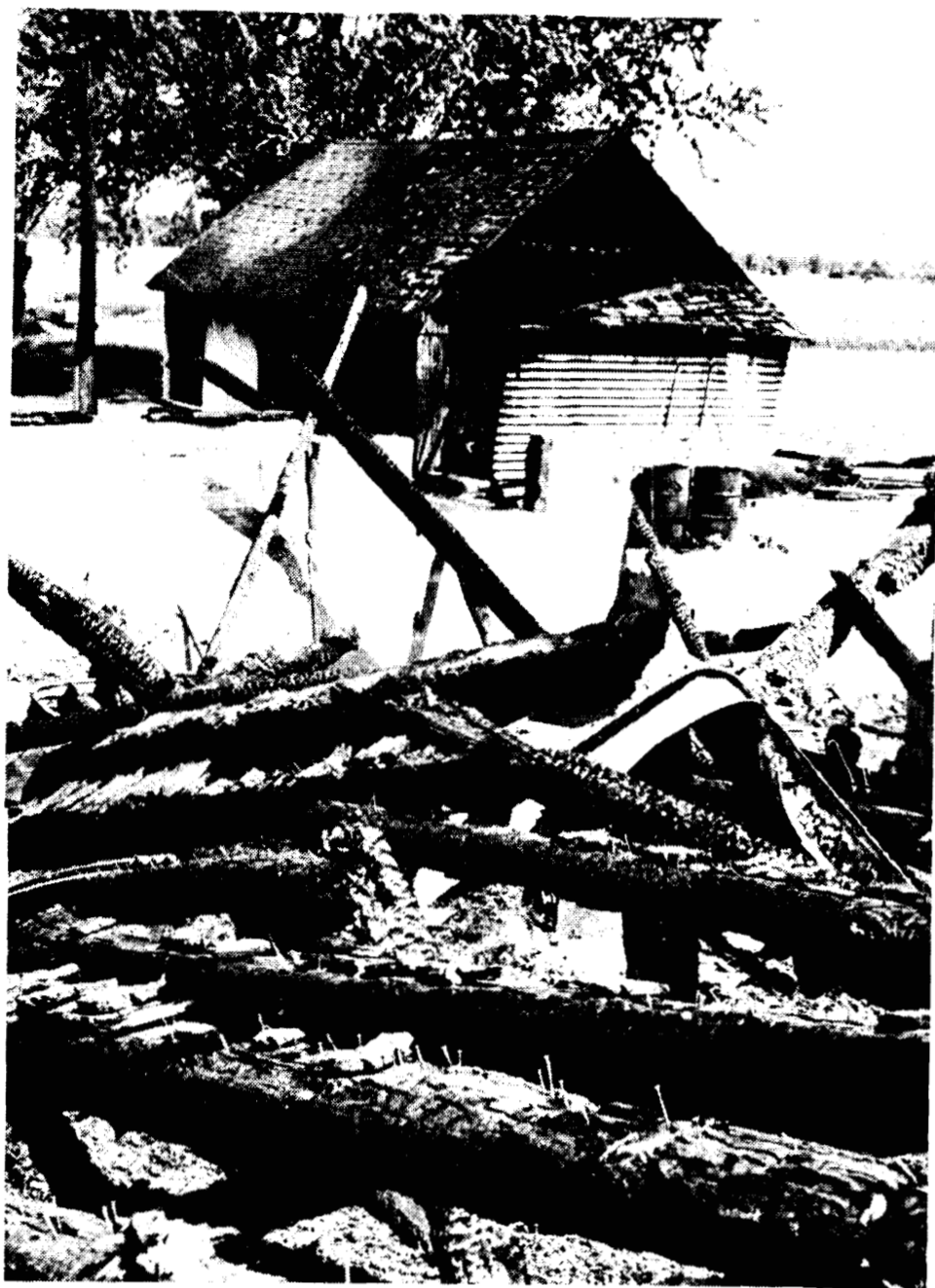
CHARRED TIMBERS that collapsed into the foundation were all that was left of the Ray and Kim Smutek barn that burned early Saturday. The fire spread to the garage in the background. It isn't considered repairable.
