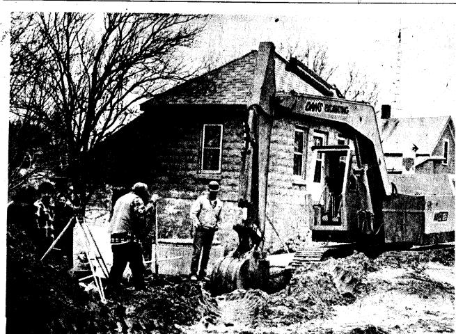
CONSTRUCTION of the \$1.8 million sanitary sewer project began in Gagetown last Wednesday with the digging of a hole and installation of a manhole on State Street at the intersection with Fifth Street. The contractor, Dan's Excavating of Utica, has a year to complete the project.
