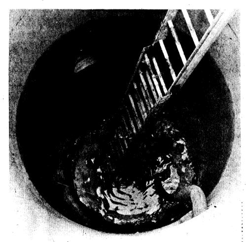
DOWN THE HOLE -- At the bottom of the 12½ foot deep: lift station Monday, digging with a shovel, was Dave Barnes. Sewer lines, not yet installed, will run into the lift station, which will then pump it into the nearest sewer
