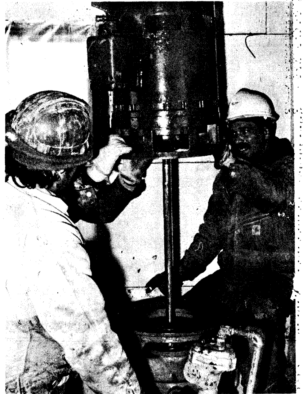
WATER WORKS -- Installation of the electric motor Tuesday, Dec. 20, was the last step in renovation of one of Cass City's two water wells, which included installation of a new shaft to run the impeller at the bottom of the well and rebuilding the motor. Lowering it into place are, from left, Mike Hedrick of Layne-Northern Co. of Lansing, contractor for the job, and village employees Ed Nizzola (hands shown) and Russ Bradley. The second well will be refurbished in January. Total cost will be about $26,000.
