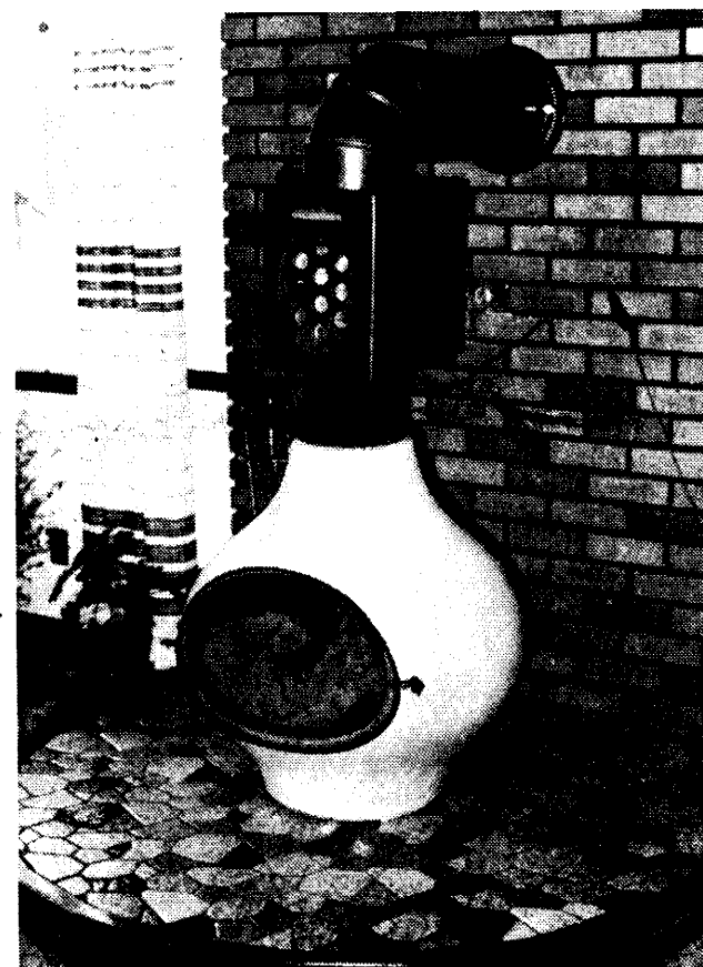
SAFE HEAT is provided by the ceramic wood burning heater in the home of Bill and Connie Klinkman on Cemetery Road, Cass City. The base consists of four inches of concrete, a quarter inch of asbestos and then ceramic tile. Behind the unit is brick, then asbestos and four inches of air space to the dry wall. The chimney walls are 10 inches of concrete. Klinkman cleans the chimney three or four times a winter. The unit is the primary source of heat in the 1,625 square foot home and burns 14-15 face cords a winter. The 200 gallon fuel oil tank was recently refilled for the first time in three years.
