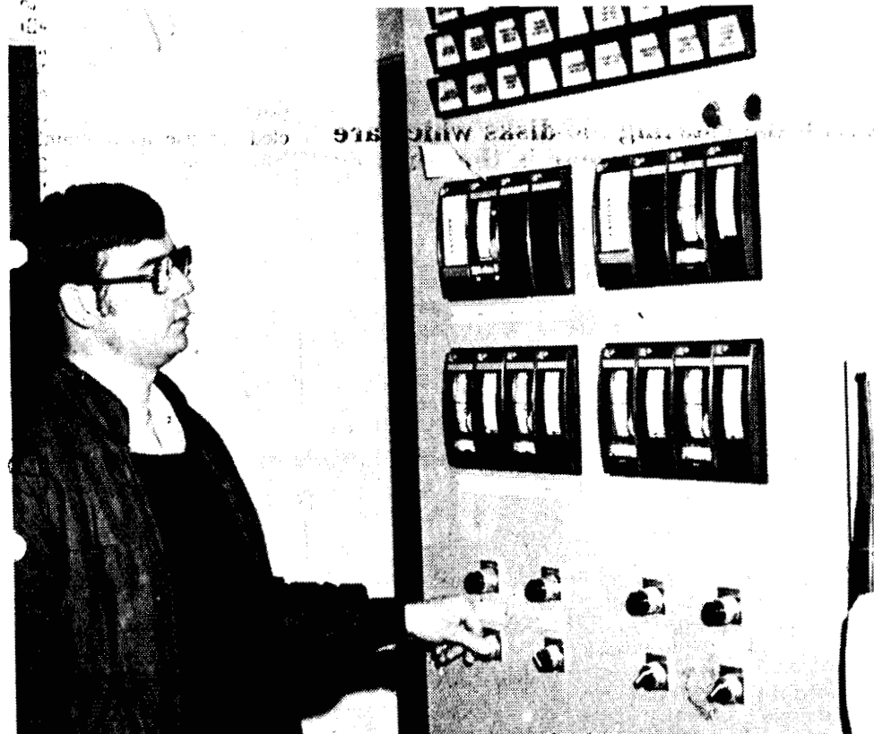
CONTROL PANEL in the main control building regulates the flow through the plant, chlorine and chemicals. At the controls is Superintendent Rick Mohr. Warning lights at the top will flash and a horn will sound if anything in the facility goes wrong.
