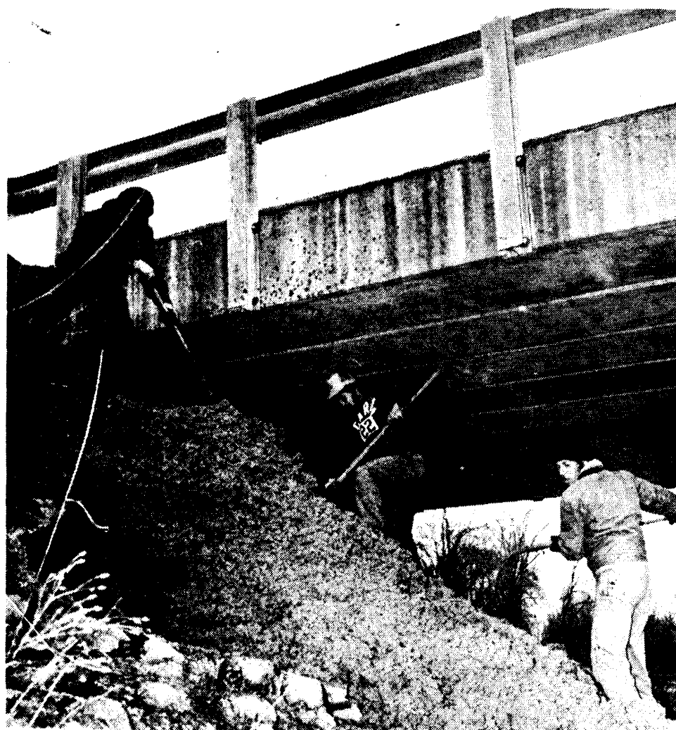
BANK JOB -- High waters washed away some of the concrete and stone riprap under the Cemetery Road bridge over the Cass River, so the county Road Commission contracted to have it repaired. Spreading the freshly poured concrete Nov. 6 were, from left, Robert Engler, Tony Quick and Mike LaFave, employed by Pat LaFave of Caro.
