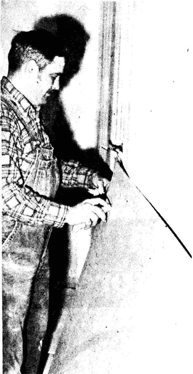
CAREFUL MEASURE -- Leo Palmer measures where to cut a piece of plasterboard, to be installed in an upstairs bedroom.
