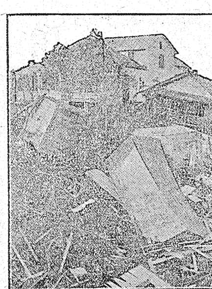
Wrecked Houses. (Kingston.)
