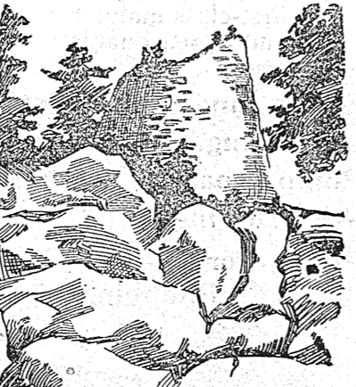
FIRST MONUMENT TO WASHINGTON IN ITS PRESENT CONDITION.
