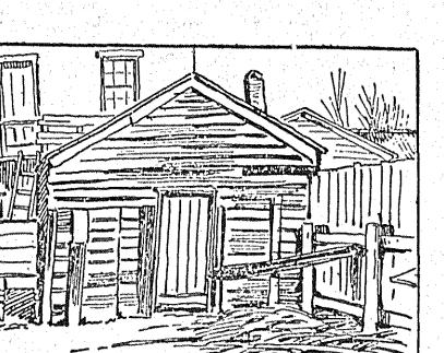
STORE AT SALEM ILL., ONCE KEPT BY LINCOLN.
